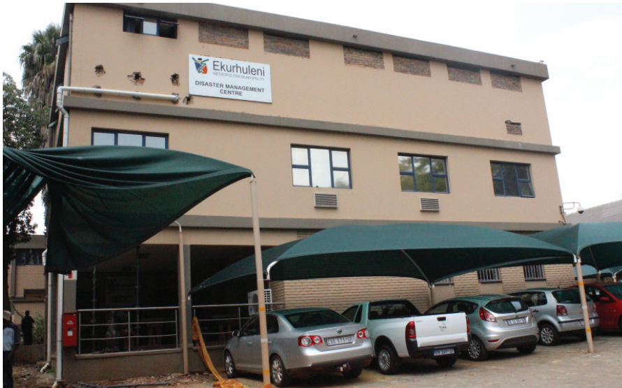
The Ekurhuleni disaster management centre is currently being upgraded
